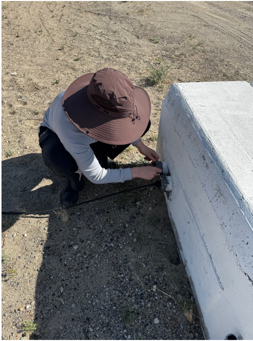
(a) Outside of the cable vault.
